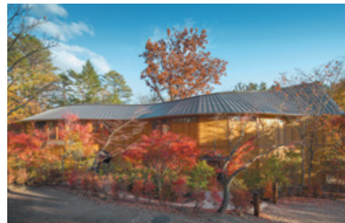
SHISHI-IWA NO 01 The prefabricated SSH No 01, by Shigeru Ban, was assembled on site, its serpentine form allowing the building to snake through trees. Picture: Hiroyuki Hirai
